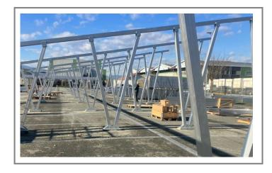
Solar PV car park canopies generate significant solar power (c.5-6kWp per 2 bays) for use at site and/or perhaps as EV charging in conjunction with a battery storage system.
