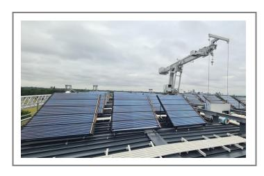
LaZer2 solar thermal is specifically designed to produce hot water.
