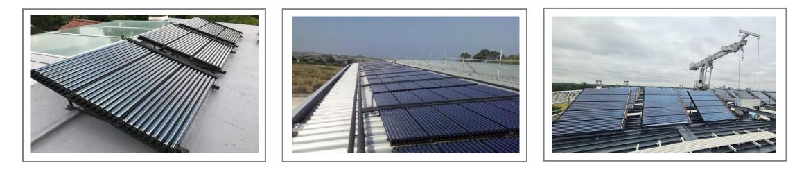
LaZer2 solar thermal is specifically designed to produce hot water.
